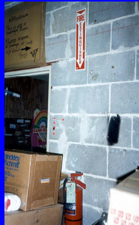
Blocked extinguisher
